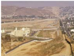
An international wastewater treatment plant
